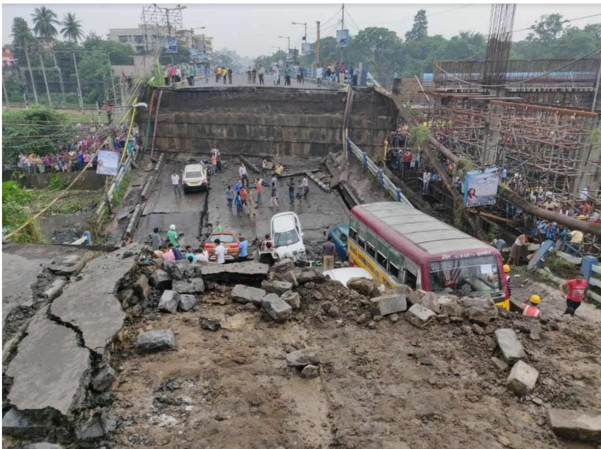
Figure 4 Kolkata bridge collapse in 2018
